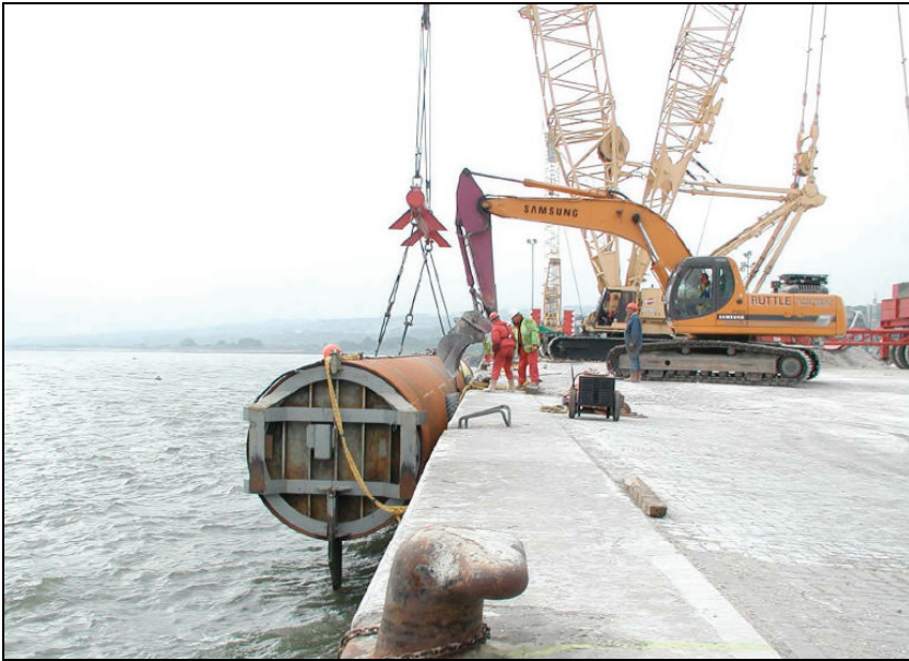
(a) Monopile being floated out to site.
