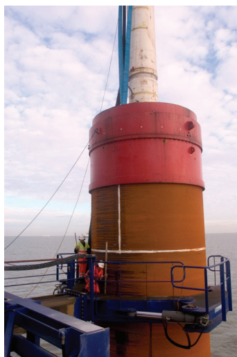
Fig. 8. Menck Pile driving hammer atop a steel pipe pile at Kentish Flats Offshore Wind Farm, UK (Courtesy: Elsam)
